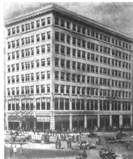
Pence Automobile Company Building.
